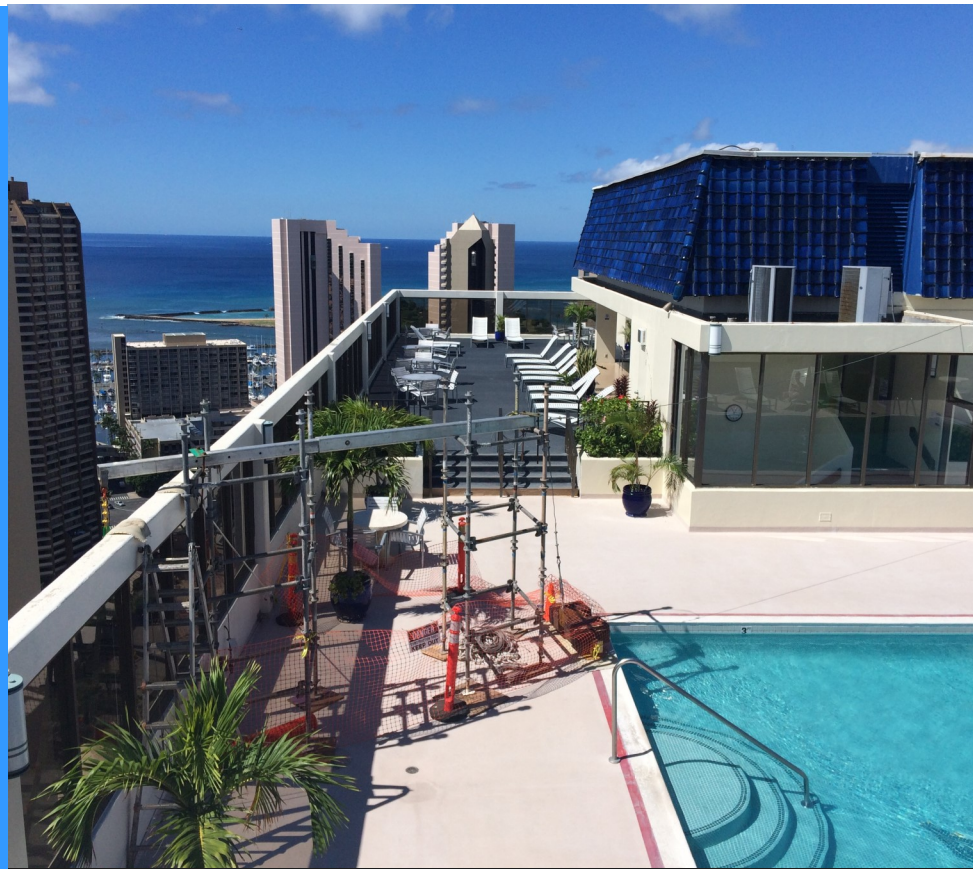
Repairs Underway on the Recreation Deck
